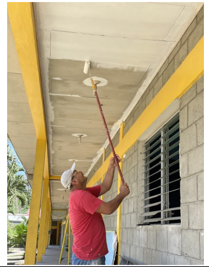
Nery painting the outside of the classrooms.
